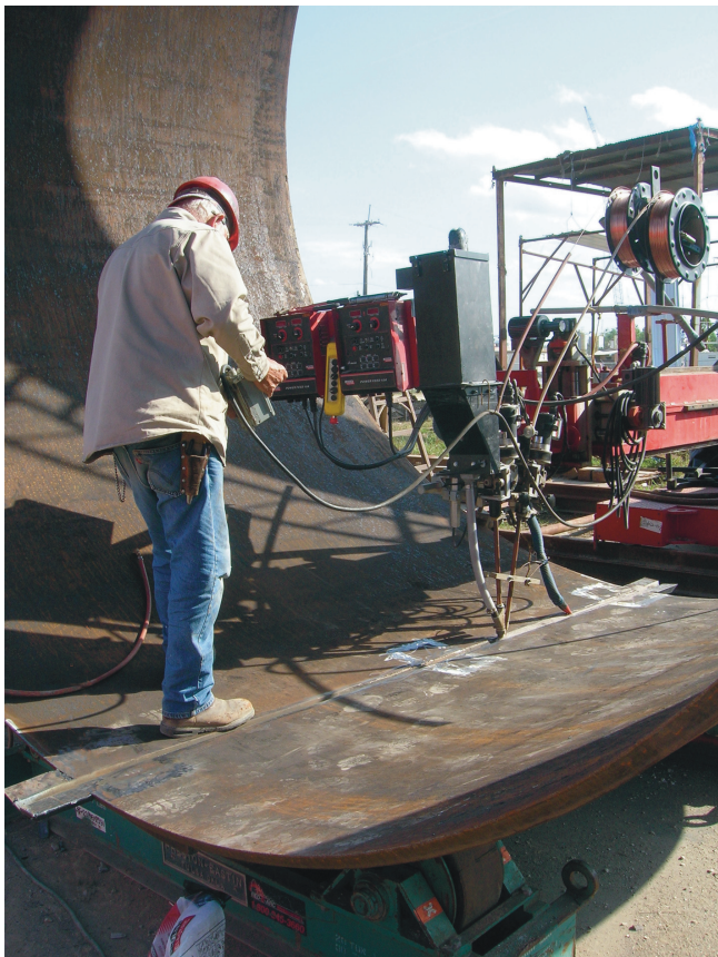
Figure 2. At New Industries, a worker is welding the inside longitudinal seam of a 1 1/2 in. thick pressure vessel using Lincoln Electric Power Wave® AC/DC 1000® submerged arc power sources in a two arc configuration.
