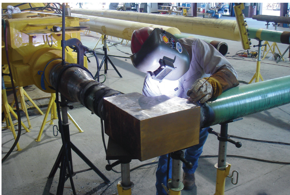
Figure 4. A New Industries welder is TIG (GTAW) welding.
